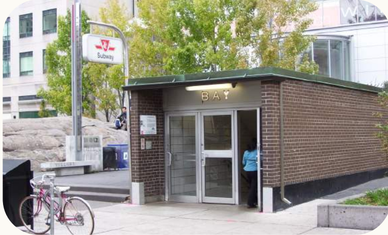
Numerous Subway Stations
