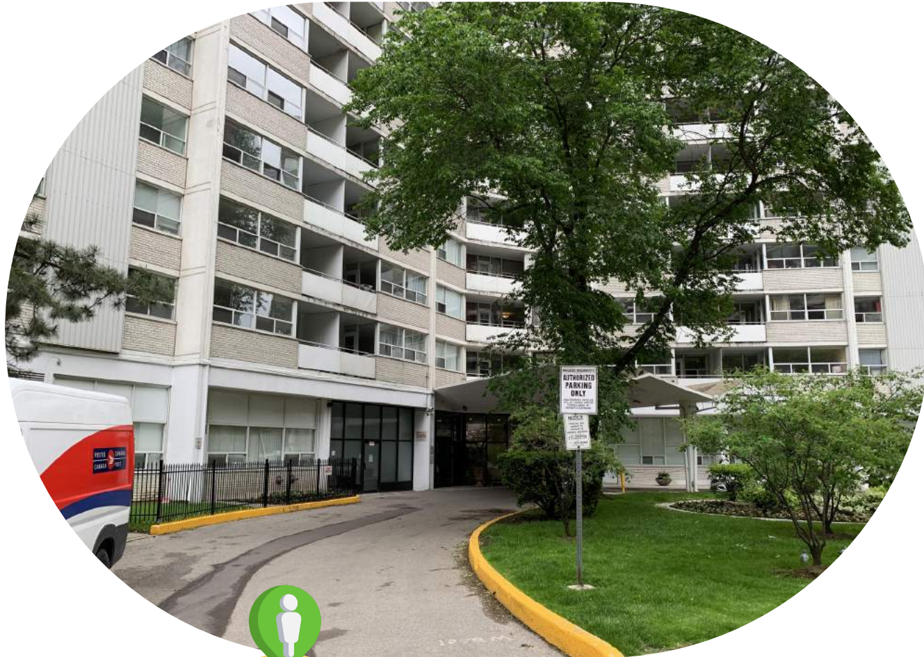
View looking south from St. Mary Street
